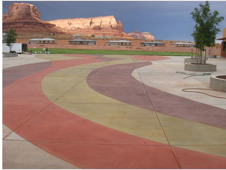
Concrete paving with oxide
