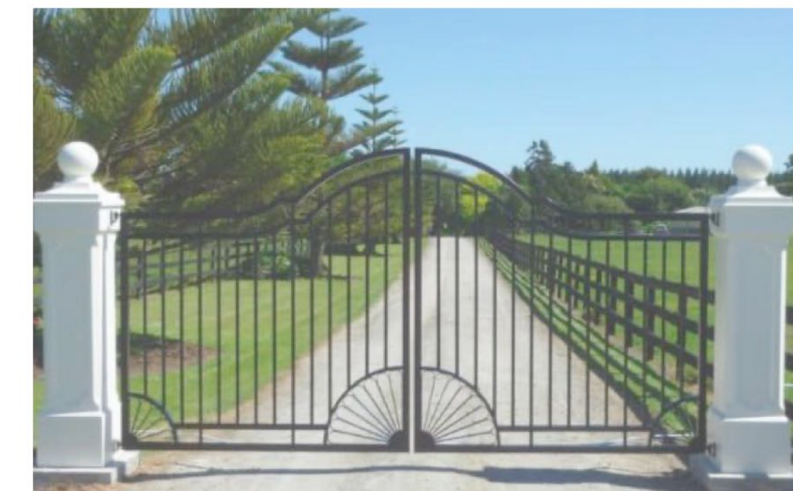
Steel curved top gate
