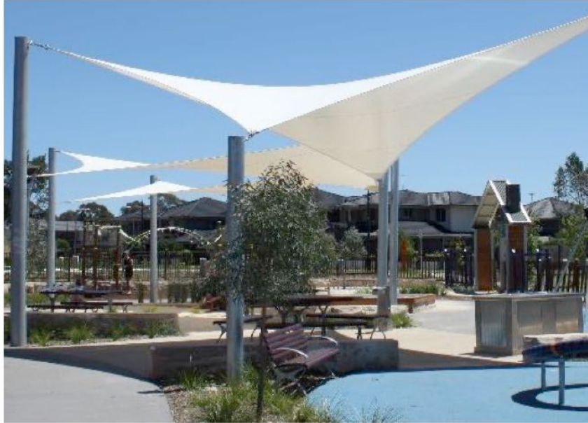
Shade sail structure
