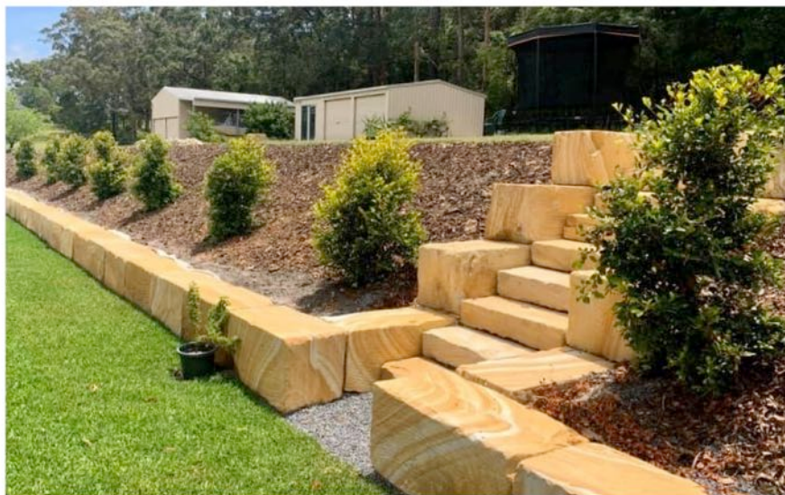
Sandstone log retaining wall
